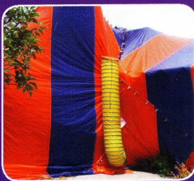
Example of duct
